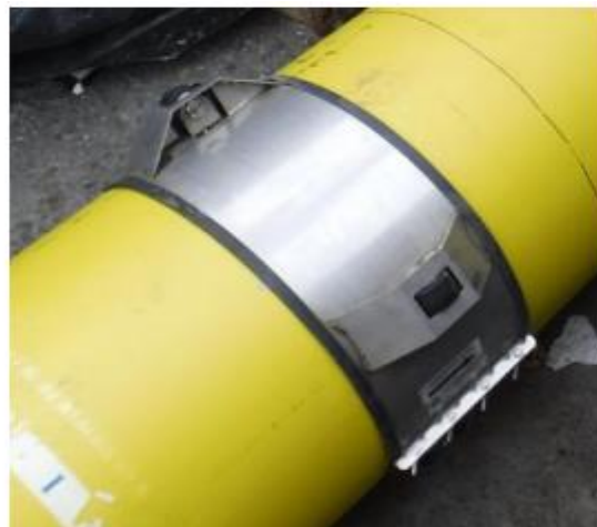
Figure 5: Final Pipeline Spacer Design installed on 630 mm PE pipe
