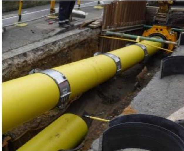
Figure 6: Spacers installed during Field Trial 1
