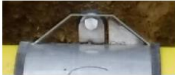
Figure 4: Spacer ramp and reinforcement gusset
