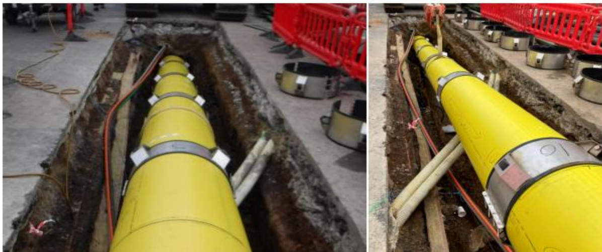
Figure 7: Spacers installed during Field Trial 2
