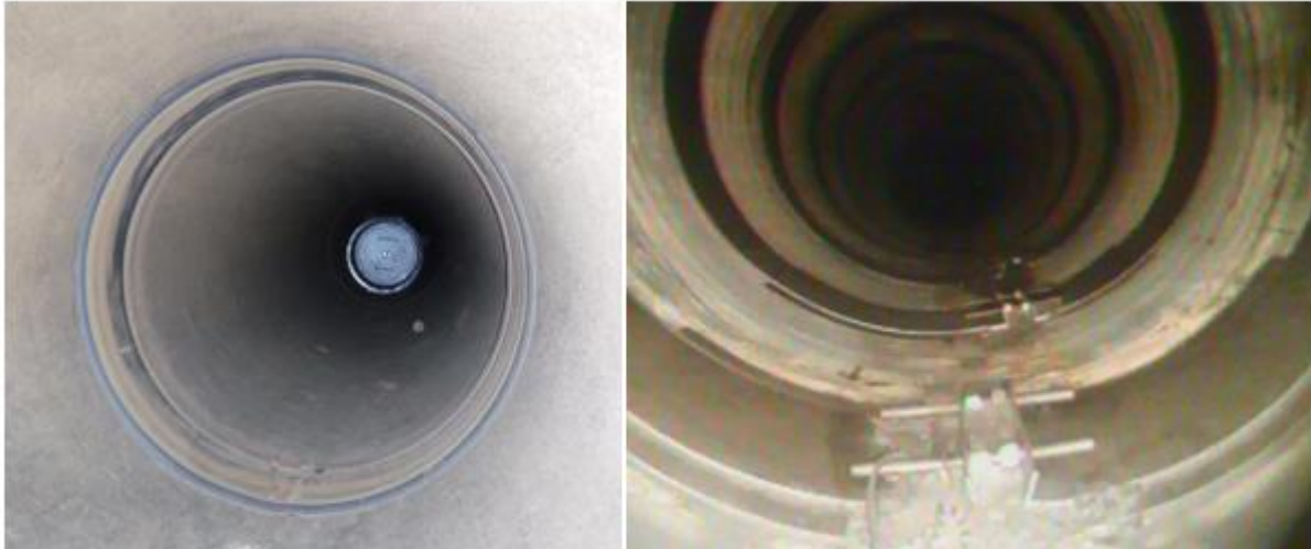
Figure 1: Weko Seals and brackets at Cast Iron Pipe Joints (Left: Wedge Spacer, Right: Large Brackets)
