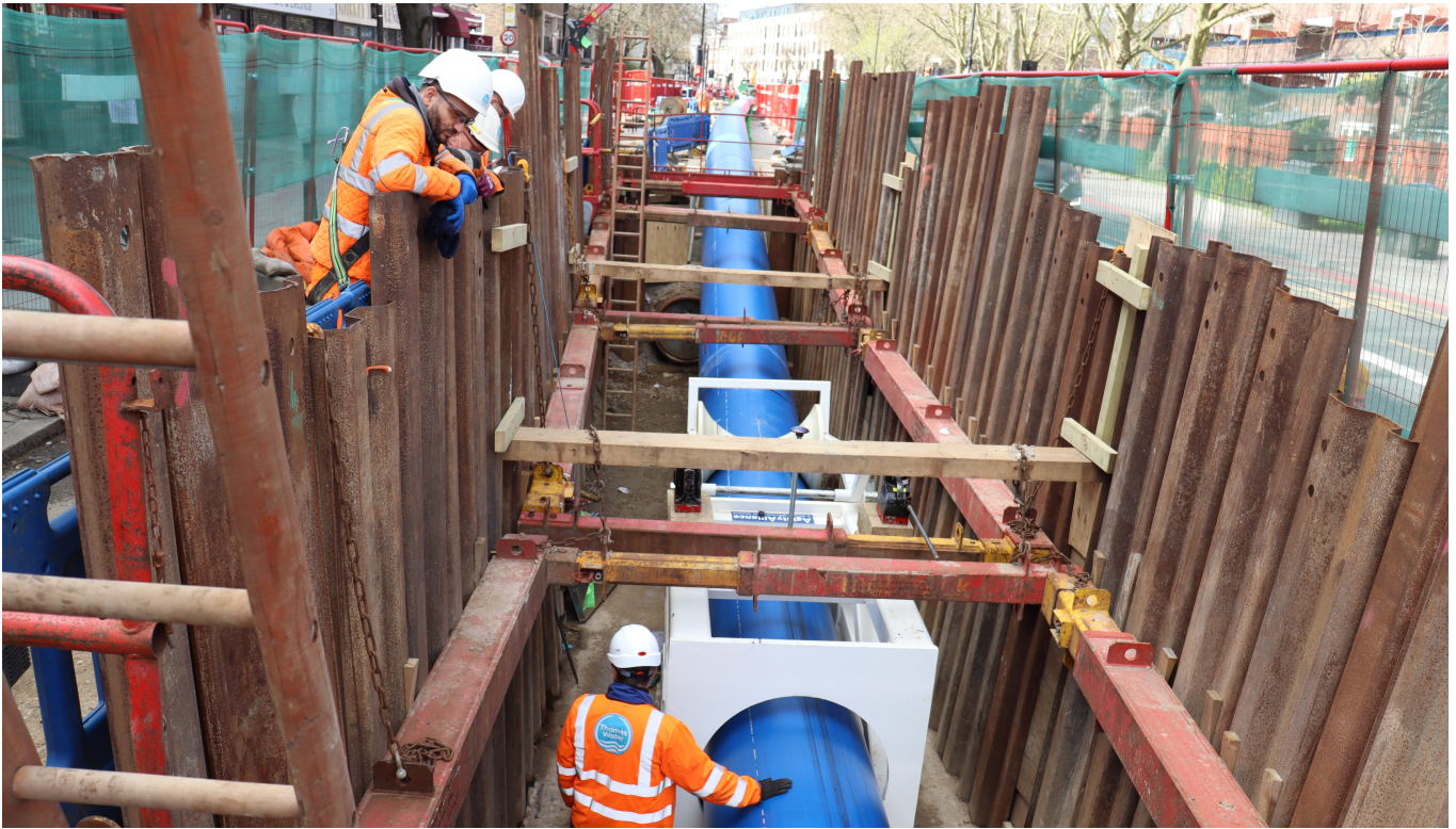
Image 3: Liner passing through die at launch pit
