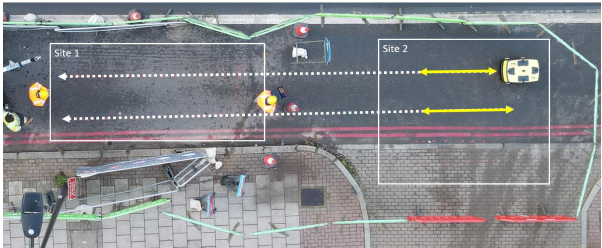
Figure 7: Comparison of paint marks in two adjacent regions that were scanned and marked out independently of each other. The white arrow shows the projection of mark-outs from site 1 into site 2. The yellow arrows highlight the paint markers placed at site 2.
