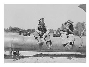
**1942-3** In the USA emergency war pipelines 'Big inch' and 'Little Big Inch' are built after oil tankers normally used for transportation are attacked by German submarines. Big Inch and Little Big Inch pipelines measure 1,254 and 1,475 miles respectively
