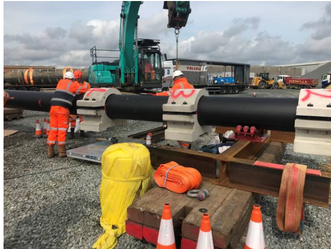
Pipe preparation in Great Yarmouth
