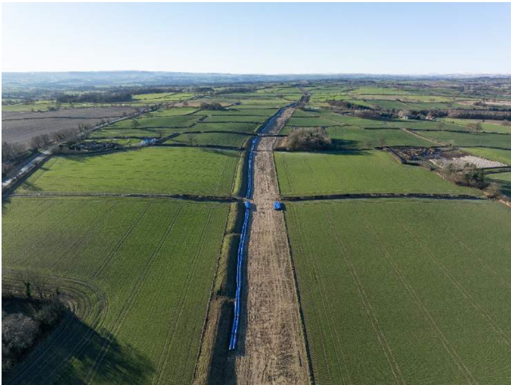
Figure 6: Pipeline Working Corridor (courtesy of Farrans)
