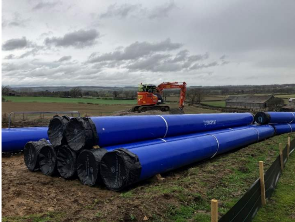
Figure 7: DN800 Pipeline Installation Works (courtesy of IDeA)
