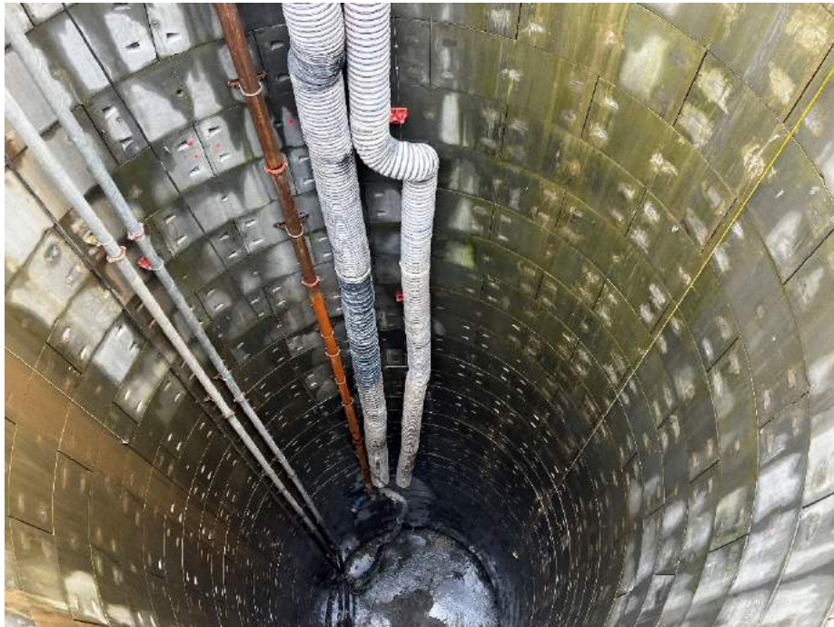
Figure 8: River Tees East Shaft Construction (courtesy of IDeA)
