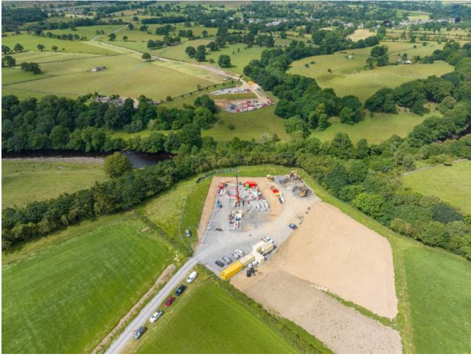
Figure 5: River Tees Crossing from East Shaft Looking West (courtesy of Farrans)
