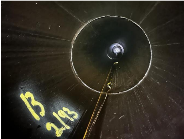
Figure 5 - Post cleaning condition after 4 runs of Air Pigging
