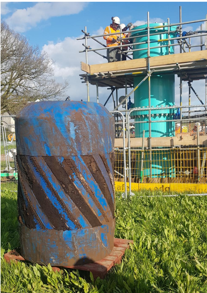
Figure 2 - Cleaning PIG condition after the first run & launcher manifold.
