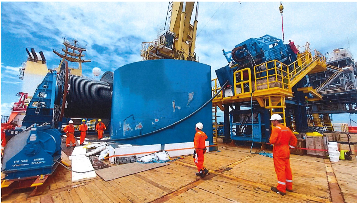
4. Installation of the first TCP with weight coating offshore Equatorial Guinea
