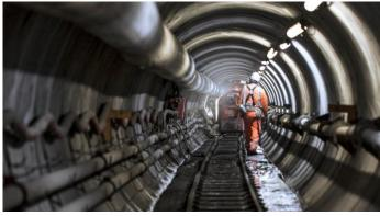
Battersea Power Station stopped generating electricity in 1983 and a new electricity substation is being built to help distribute power to homes and businesses across the new neighbourhood. The substation will connect to the existing electricity network via the Battersea Cable Tunnel.
